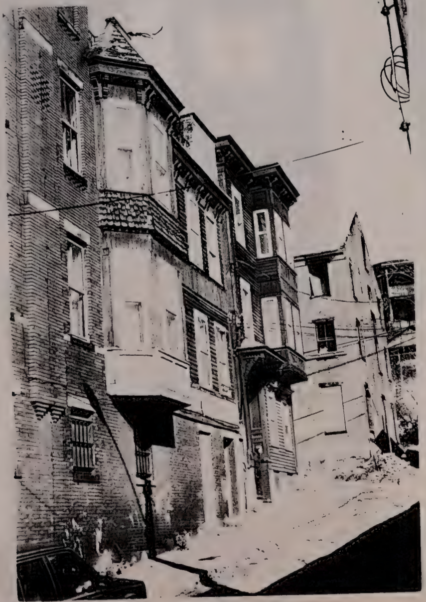
↑ Side wall, #207-217 Main St.
